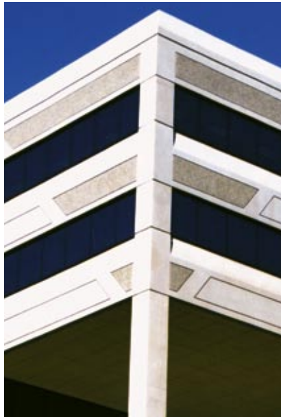
Textures and varying depths added visual interest to the structure. The panels feature both rough, exposed aggregates and a smooth, sandblasted appearance.
